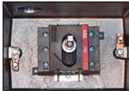
Internal view showing DIN rail mounted ABB OT63F3 non-fusible, heavy duty, disconnect switch with dual grounding lugs and actuation shaft.
