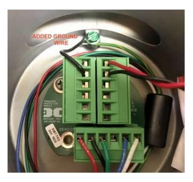
Note the added ground wire used to comply with the instruction found in the manual. A similar wiring scheme should be used if the DM700 and PI700 are used either without the condulet or with one of the optional Remote Access Modules (RAM) available for these ITM's.
