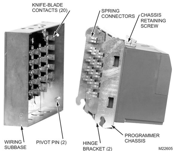
Fig. 3. Mounting the programmer on the subbase.
